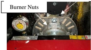
Figure 25 - Riello Burner Tube & Mounting Bracket
