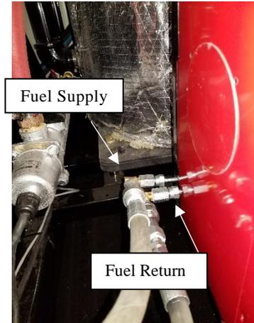
Figure 22 - Fuel Connections
